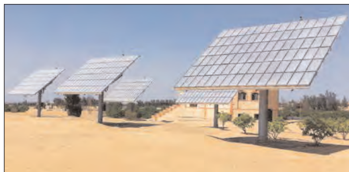
Figure 4. Installation of SOITEC CPV technology at Wadi El Natrun, Egypt.
