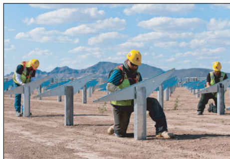
The Agua Caliente solar project under construction.
