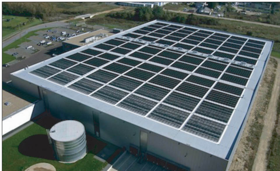
The warehouse of motorcycle accessories distributor Parts Europe GmbH of Konz, near Trier, bearing Solyndra's largest installation in Germany.
