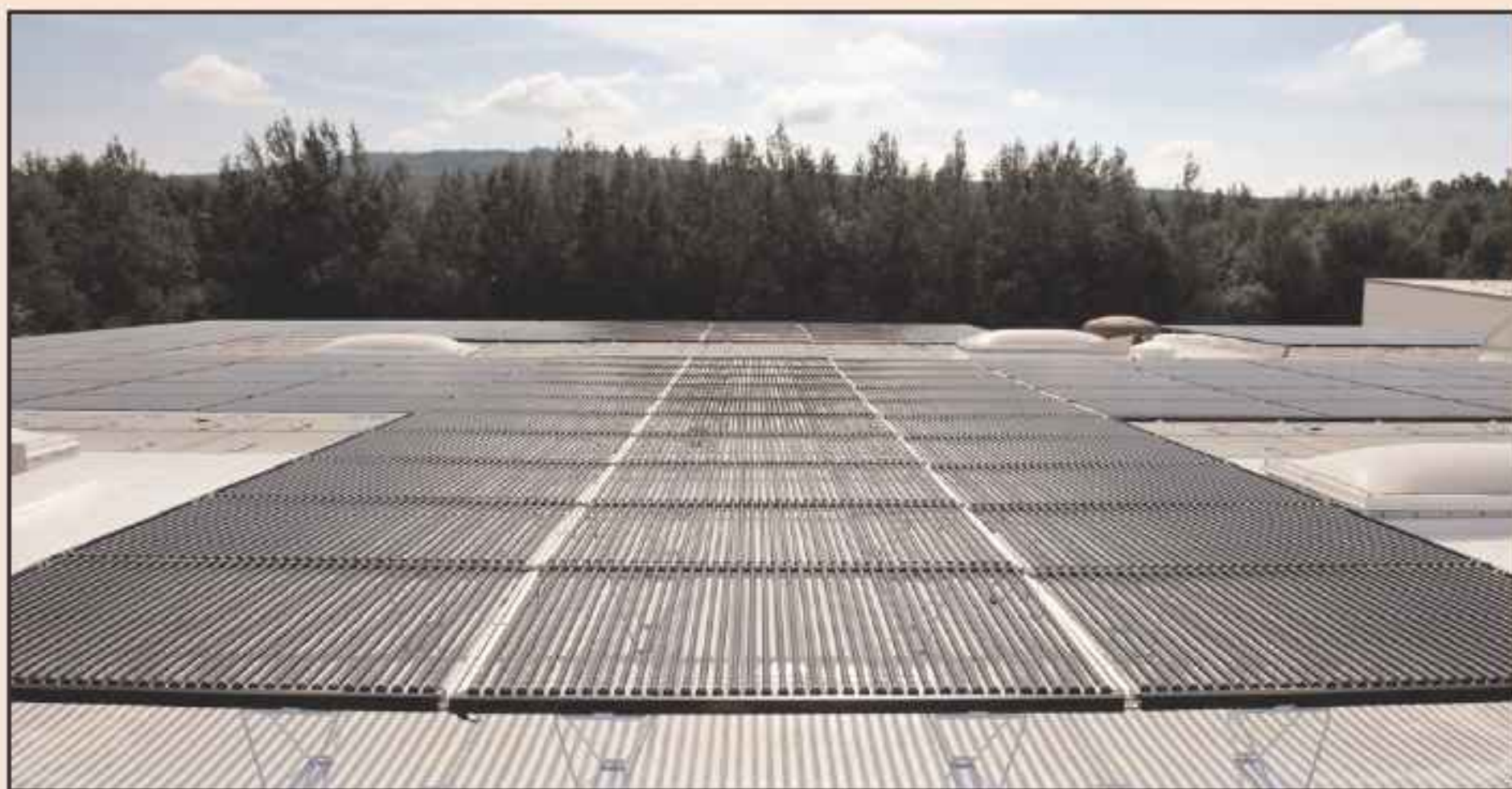
Solyndra CIGS photovoltaic arrays on alwitra roofing.
