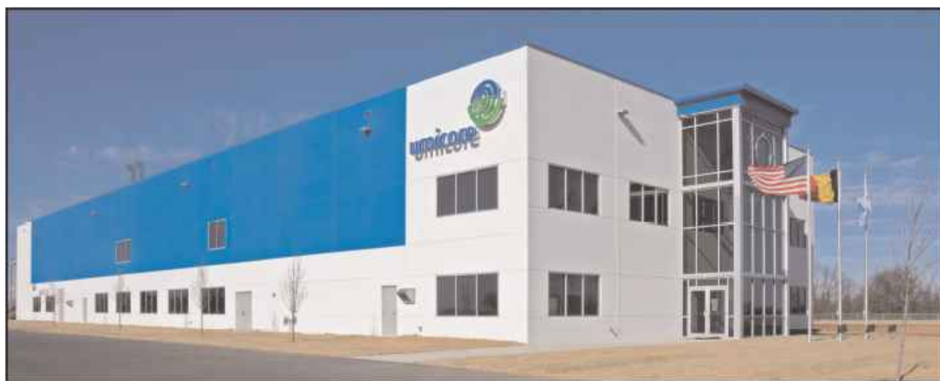
Side view of Umicore's new facility for germanium wafers in Quapaw.
