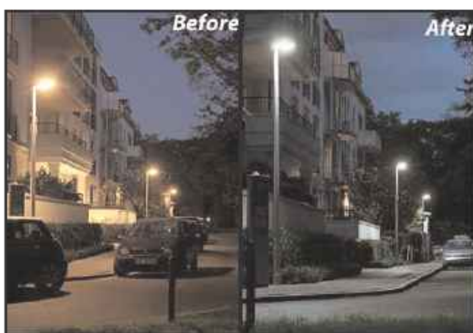
Street in Bremen before (left) and after (right) replacing compact fluorescent lights with LED fixtures.
