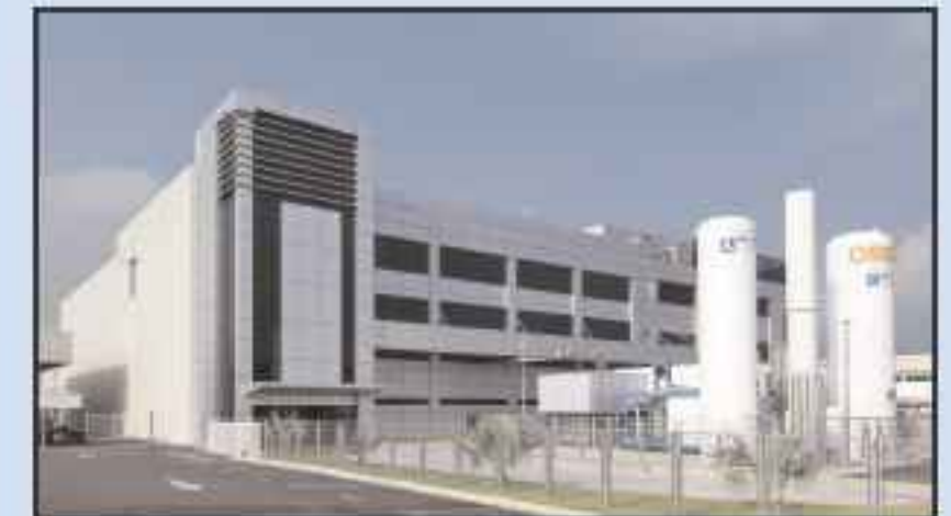
p65 Osram Opto inaugurates its first LED chip fab in Asia, at its LED chip packaging site in Penang, Malaysia.
