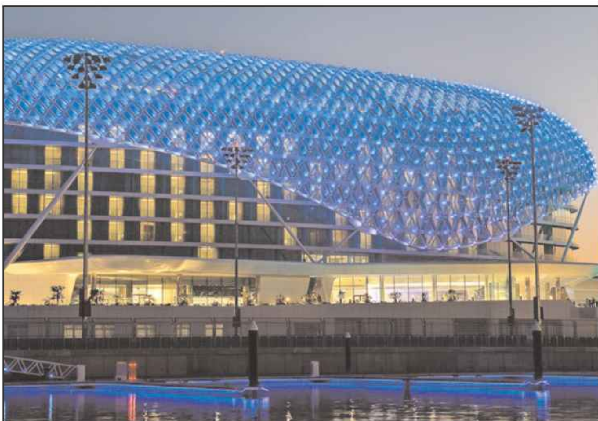
Figure 1. LED lighting at the Yas Hotel, Abu Dhabi (courtesy Enfis Ltd).
