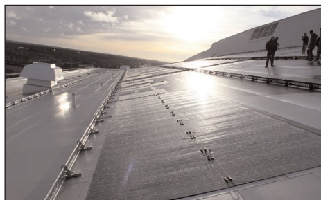
Solar panels covering the Tele2 logos on the roof of the new multi-venue Tele2 Arena in Stockholm.
