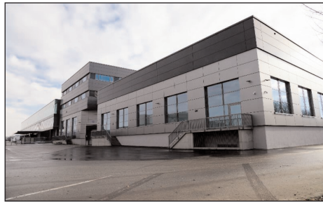
Completed building at EVG's HQ.
