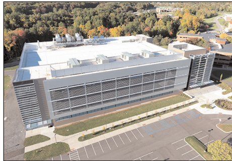
The NY-PEMC facility in Utica, upstate New York.
