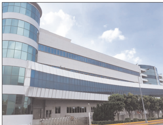
The new Tongluo factory for automotive LED components.
