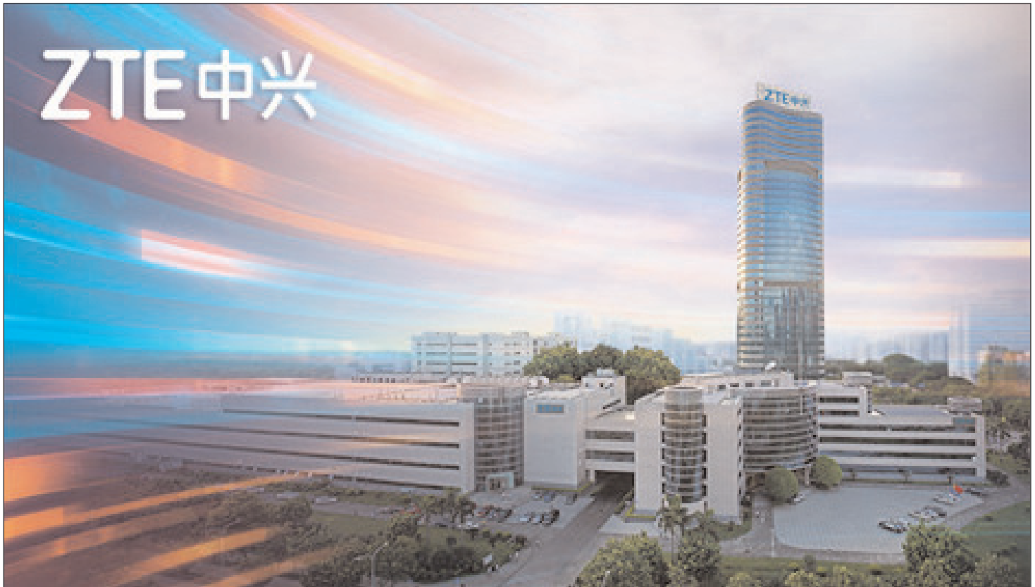
ZTE's headquarters in Shenzhen, China.
